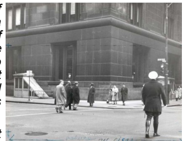
Entrances to public toilets at LaSalle and Washington Streets in Chicago prior to 1955. These entrances no longer exist.
